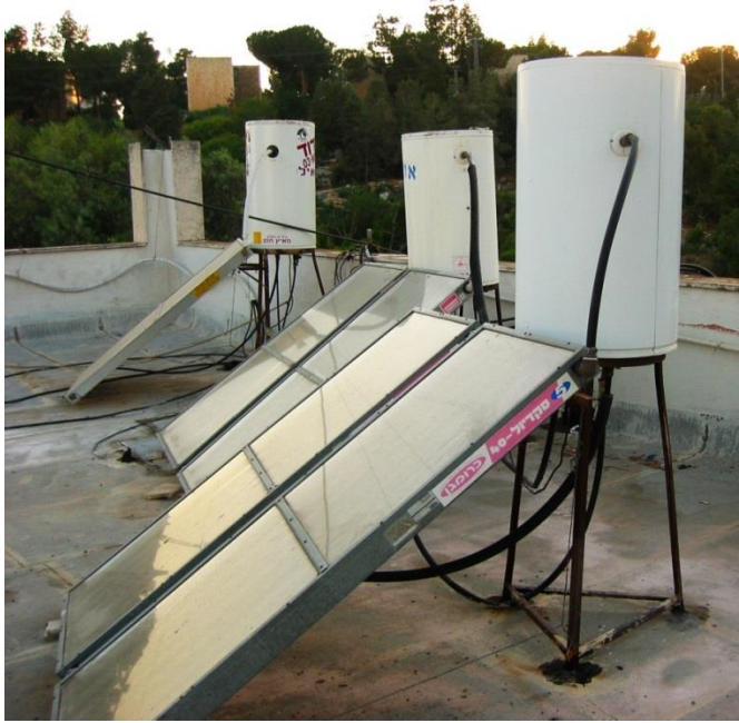
Passive, direct thermosiphon solar water heaters on a rooftop.
